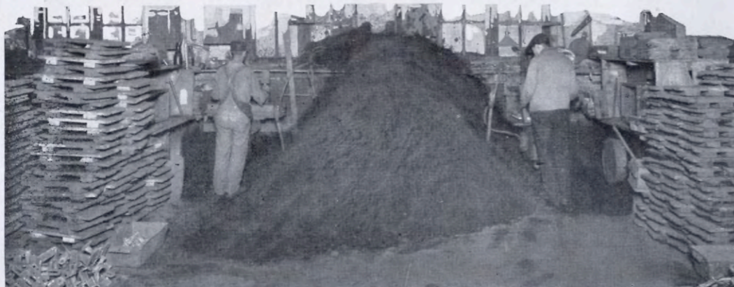
For big production use the "American" Sand Cutting Machine. It cuts, mixes, cools, and piles to perfection.
